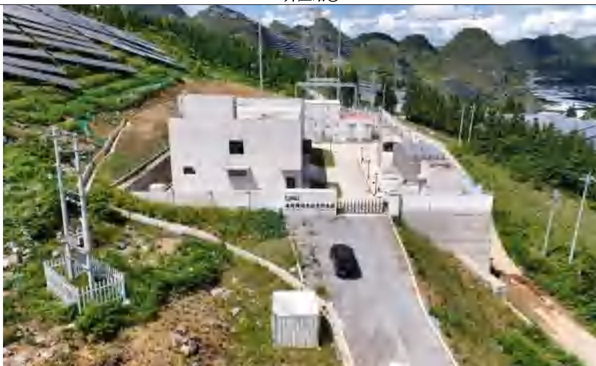
升压站现状②
