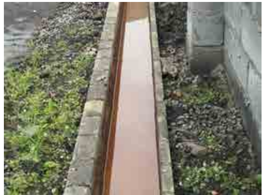
矸石场截排水沟
